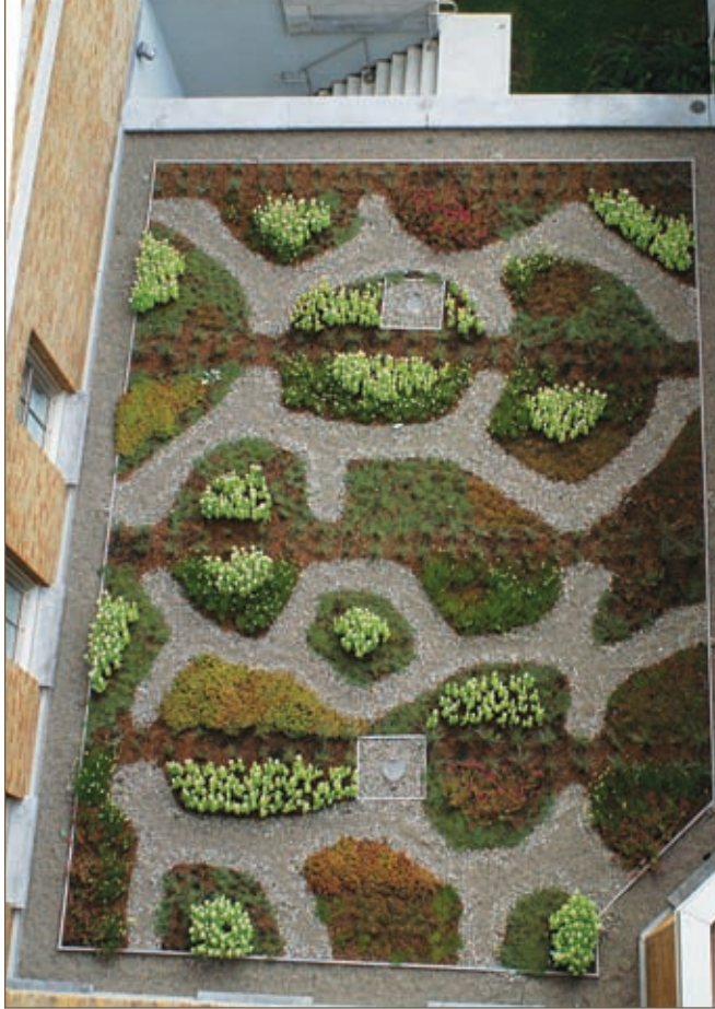
Looks can be deceiving: The green roof at St-Mary's Health Centre in Montreal looks semi-intensive, but is actually extensive.
