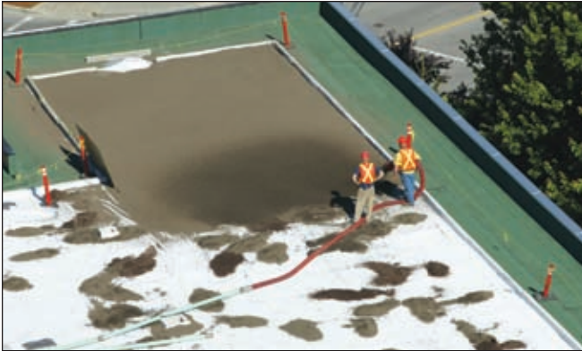
Recently introduced blowing equipment delivers soil from ground level to the roof, making the promise of green roofs more accessible.
